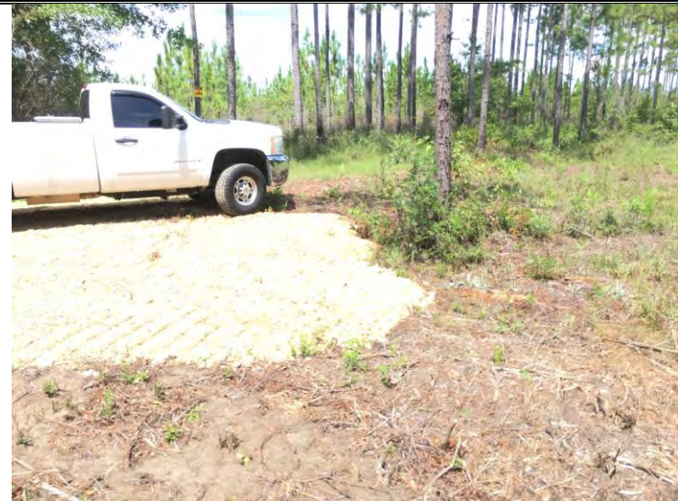
South side of improved lime rock access road.
