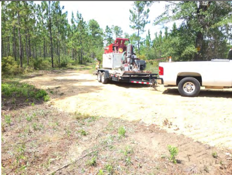
Mud machine and pump on trailer being mobed on site.
